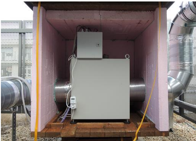
Installation of PET-02 in air ducts in a nuclear medicine facility
