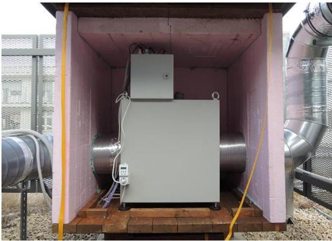
Installation of PET-02 in air ducts in a nuclear medicine facility
